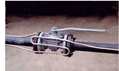
Bare Tube Tracing
